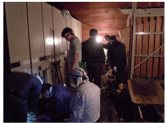
Fig.1 Debris Removal in 1F Art Storage Areas (April 26, 2011, photo: author)
