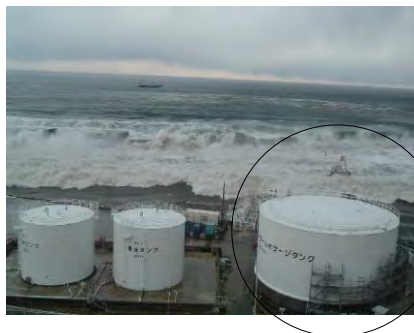
Fig. 22 Buckling failure of a water tank due to the water pressure (Provided by TEPCO)
