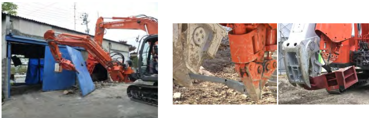
(a) Removing the doors of a damaged warehouse
