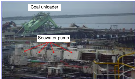
(a) Damaged coal unloader and sea water pump.
