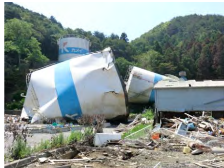
Fig. 21 Tanks washed away by tsunami
