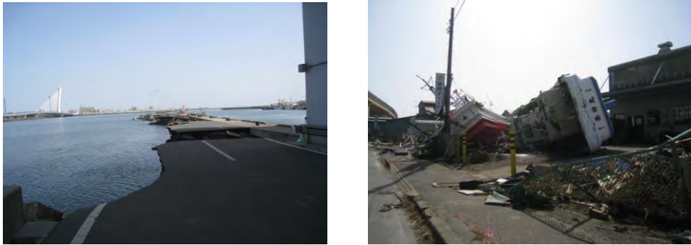
Fig.3 Damages to Hachinohe port
