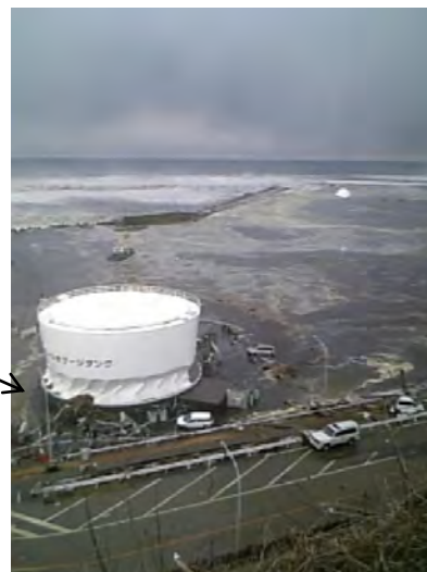
Fig. 21 Tanks washed away by tsunami
