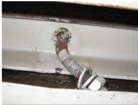
Fig. 12 Elongation of a hook bolt
