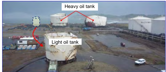
(b) Damaged light and heavy oil tanks.
