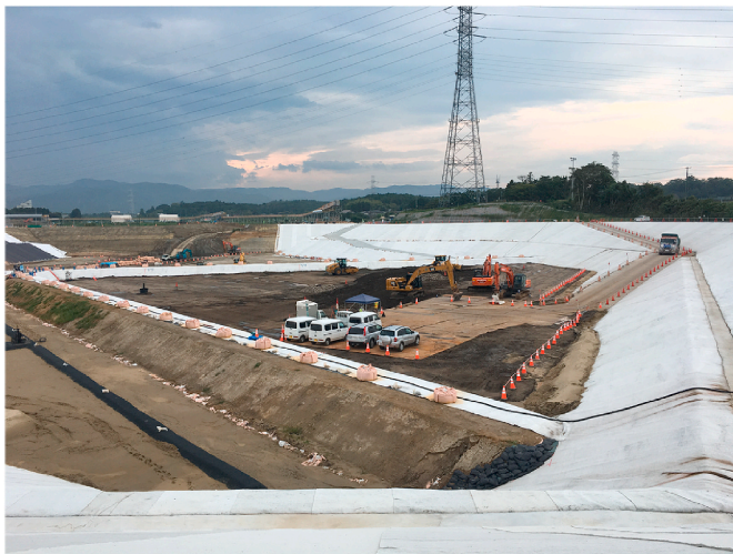
Construction work on a facility for containment of radioactive soil. Okuma-Machi, Fukushima. Photo: Miranda Schreurs, 30 August 2018.
